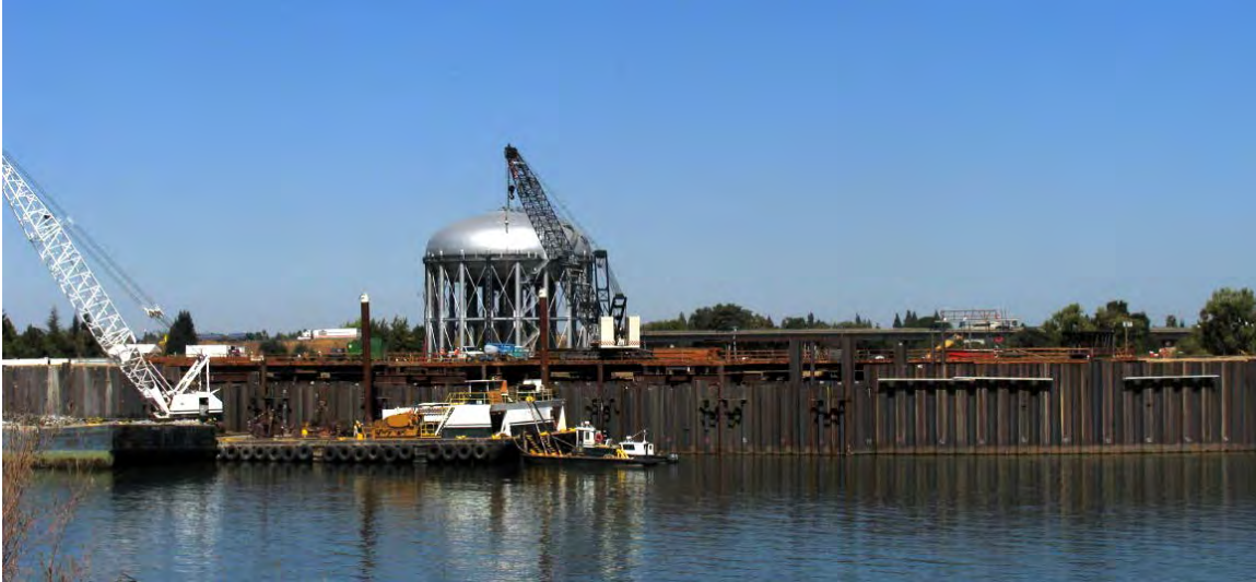
Figure ES-3. Freeport Diversion under construction September 2007
